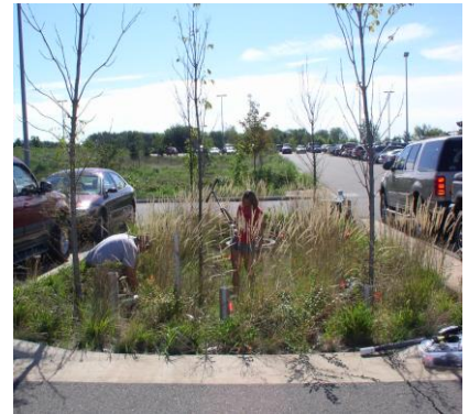
Typical biofiltration practice (Cottage Grove, MN, courtesy B. Asleson)
