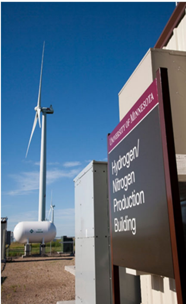
Wind to Hydrogen/Ammonia Production Project at West Central Research and Outreach Center
