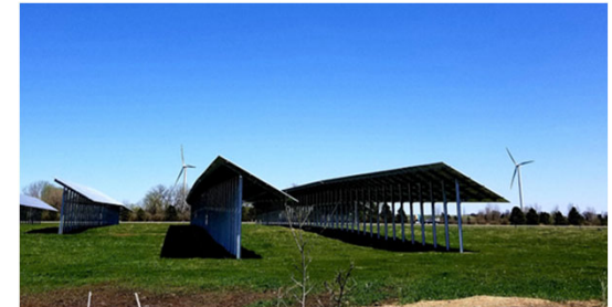
Solar Array at UMN Morris elevated to allow cattle to graze
