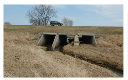
Problem – culverts can disconnect floodplains by confining water flow under a road, leading to detrimental erosion and sedimentation, increased risk to infrastructure and disrupted fish and animal movement.
