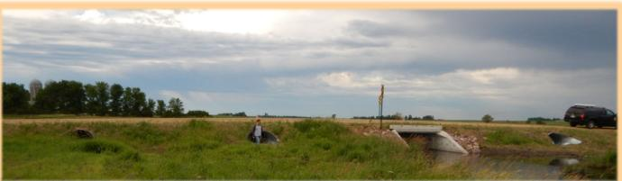
Solution – road-stream crossings that allow for water and sediment movement both in the stream and across the floodplain with floodplain culverts.
