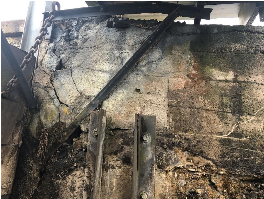
A portion of the west dam abutment wall proposed to be replaced.
