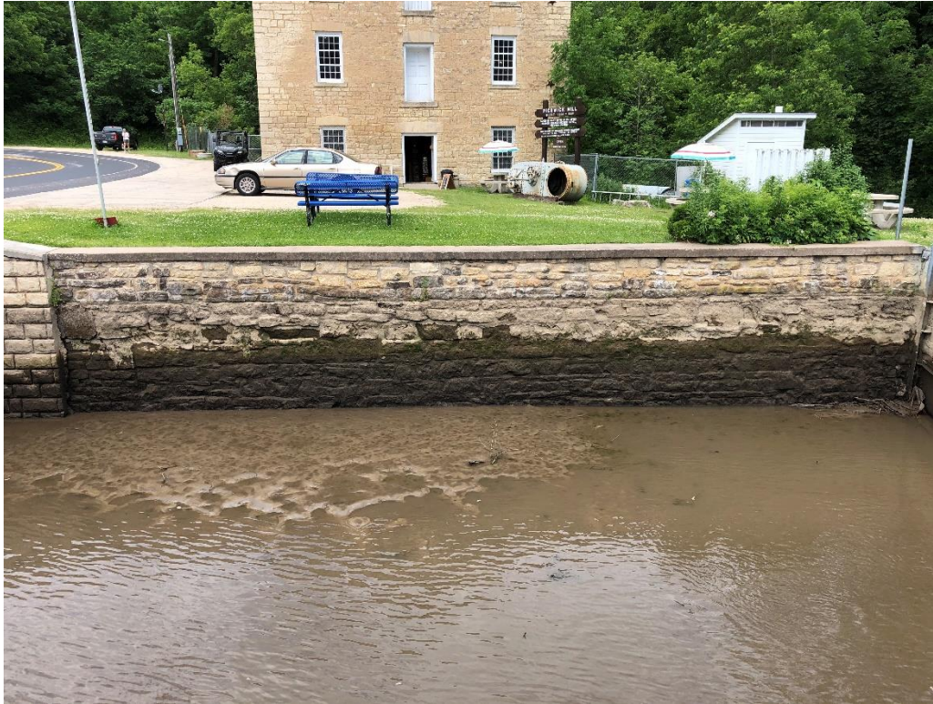
West chute wall proposed to be excavated, tuckpointed, and a clay embankment and drain tile installed on the land side of the wall to address leakage through wall.
