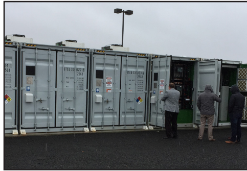
exterior of flow batteries
