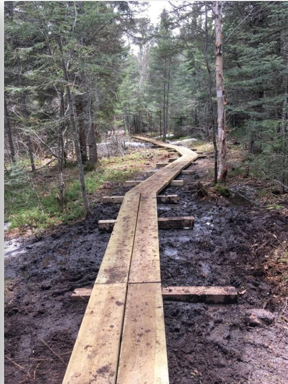
Installed near Oberg Mountain, 2019.
