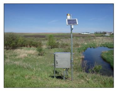
Example of installed wetland hydrology monitoring station.
