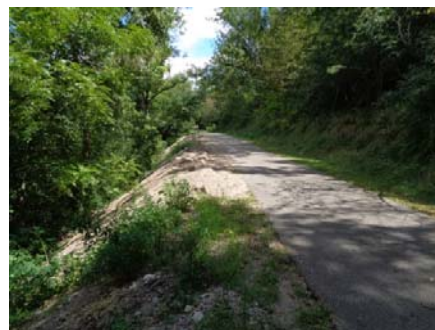
Slope failure releases large sediment loads into the Cannon River. The Cannon River ((not visible) is at the base of the slope on the left.
