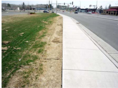
Effects of de-icing agent on the vegetation of the road shoulder (photo courtesy from Stenlund, Dwayne)
