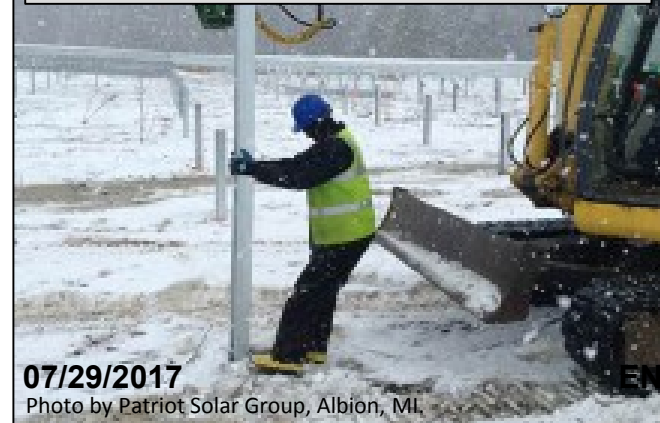
“Challenging” - ground-mount installation
