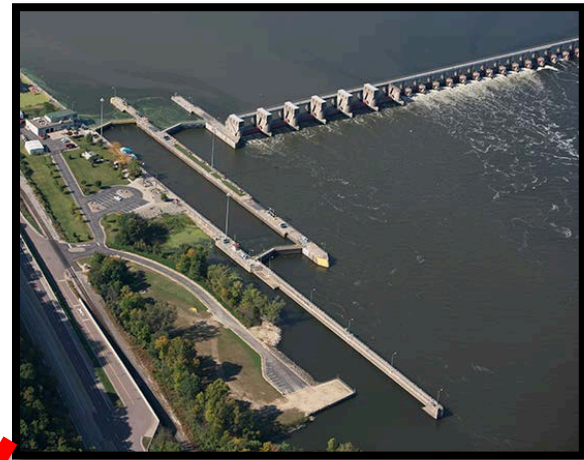
Lock and Dam #5
