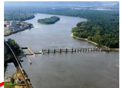
Lock and Dam #8
