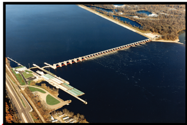
Lock and Dam #5
