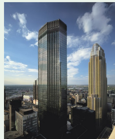
IDS tower: 50.000 m 2 of windows that could generate electricity ENRTE ID: 135 E (Image from ids-center.com)
