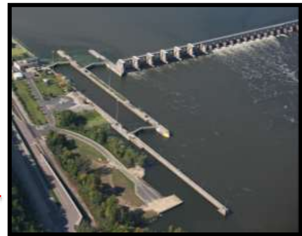
Lock and Dam #5
