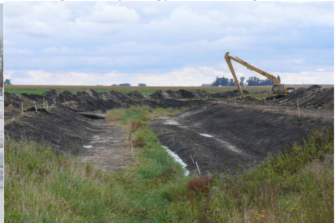
Two-stage ditch hydrology/nutrient mitigation
