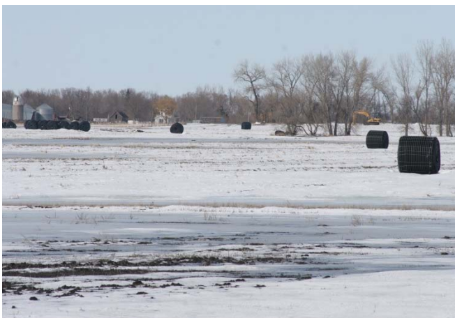
Tile set for installation
