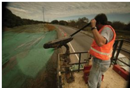
Hydroseeding will be applied to the upper part of the bank
