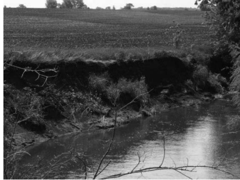
Streambank erosion LeSueur River Watershed
