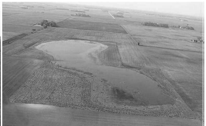
Tile Outlet to Restored Wetland, Seven-Mile Creek
