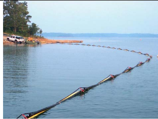
Figure 3. Linear diffuser deployment before sinking
