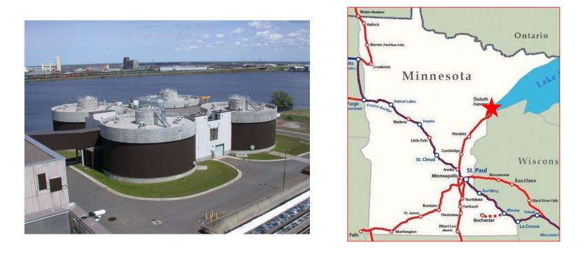
Anaerobic digestion is commonly used to treat sewage sludge, but high temperature anaerobic digestion is rare. An exception to this rarity can be found in Duluth (shown above), where high temperature anaerobic digestion has been successfully used for decades.
