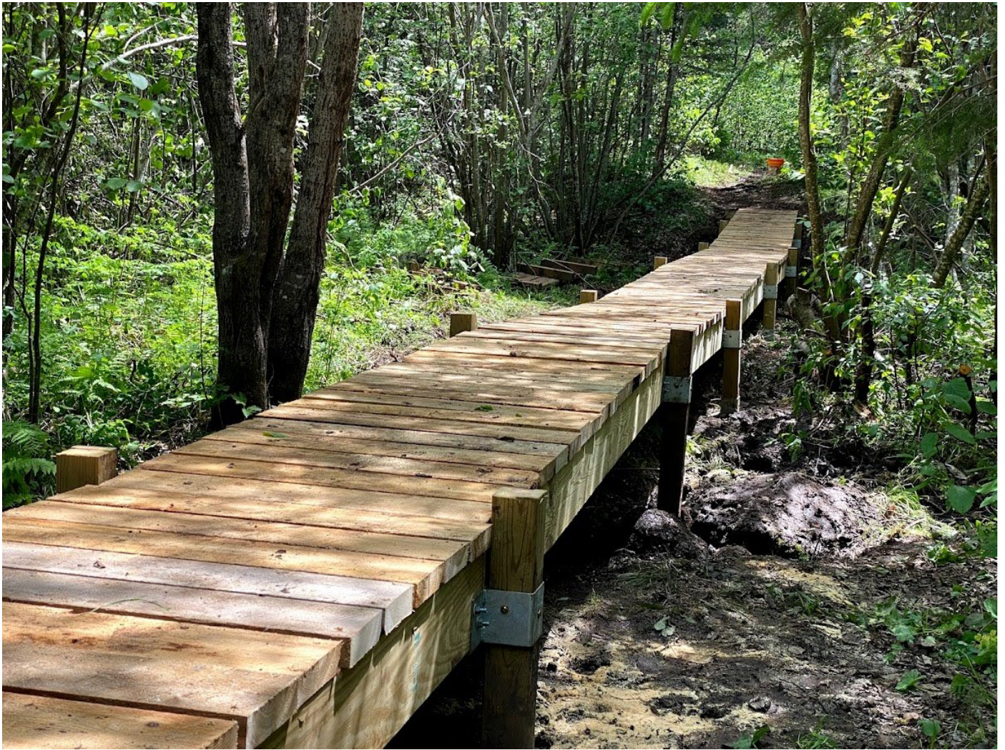
Photo: Elevated boardwalk using bog pans on Poplar River Puncheon Project
