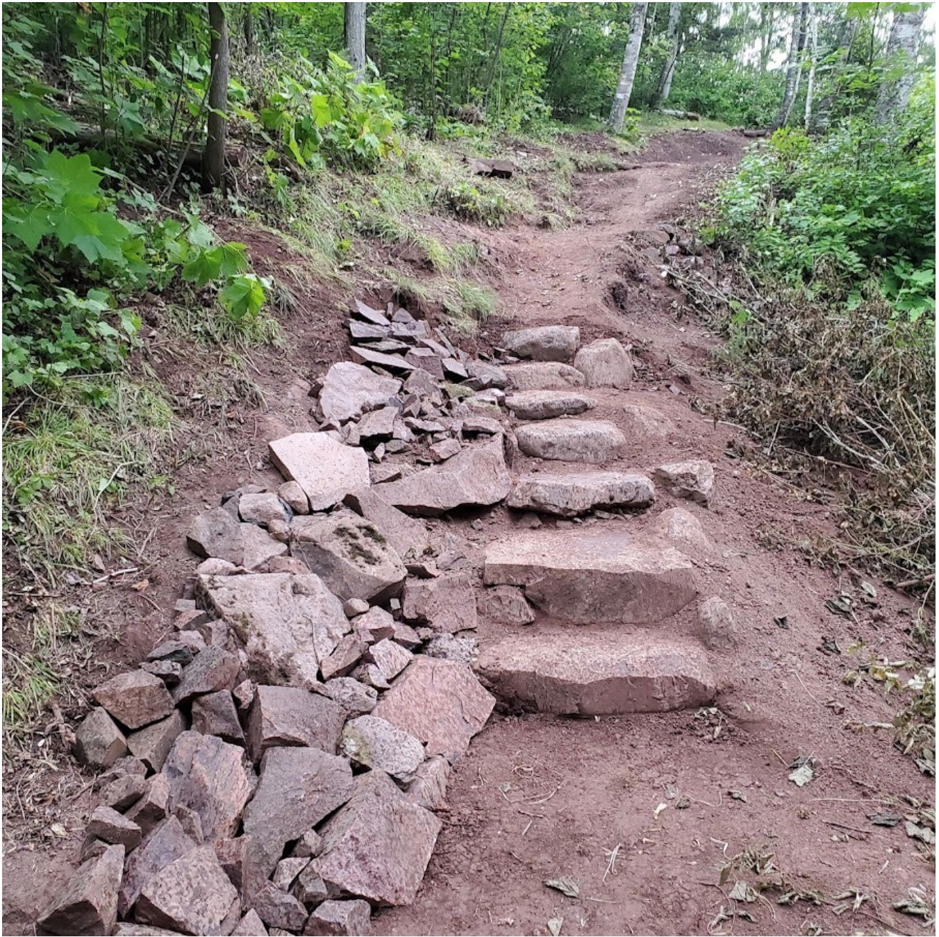
Photo: Stone steps and erosion control along descent to new bridge along Split Rock River Loop.
