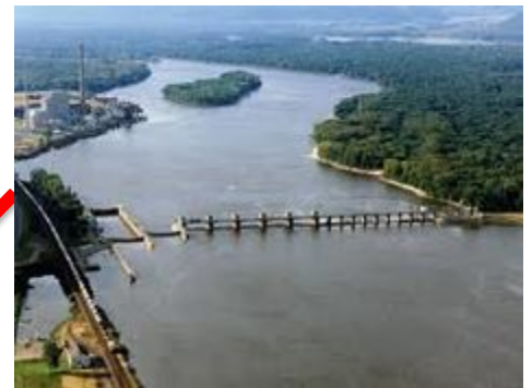
Lock and Dam #8
