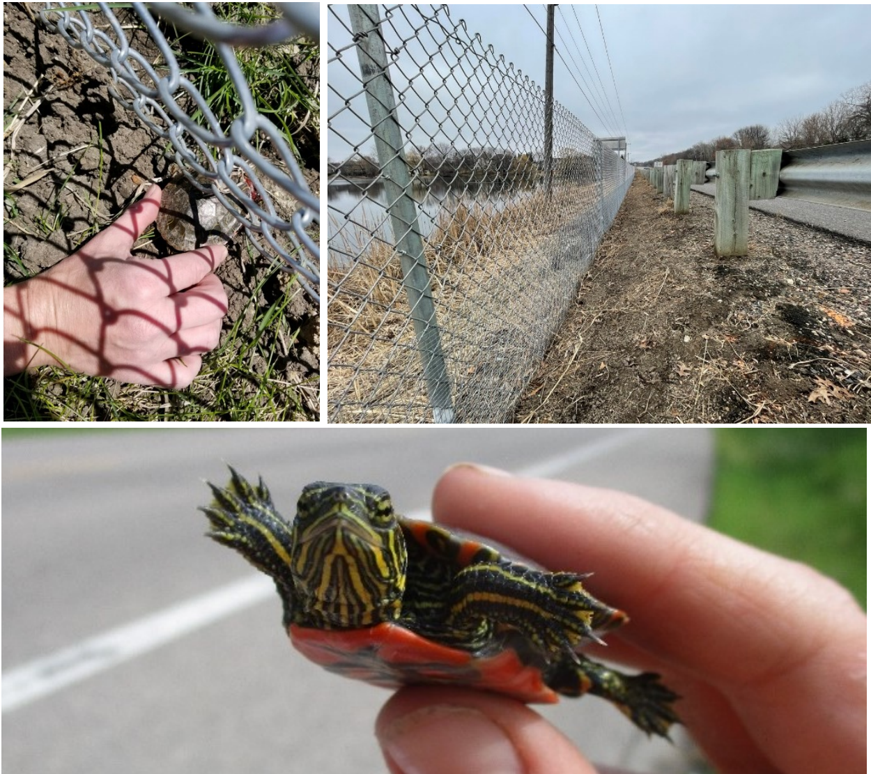
Figure 4. Top left: Small (i.e., juvenile turtles less than 2 inches in width) are able to fit through standard chain-link fence mesh and access roadway. Top right: Hardware cloth was retrofitted onto the existing chain-link fence at 3 of 4 treatment sites in 2021. Bottom: Small painted turtle found on roadway.
