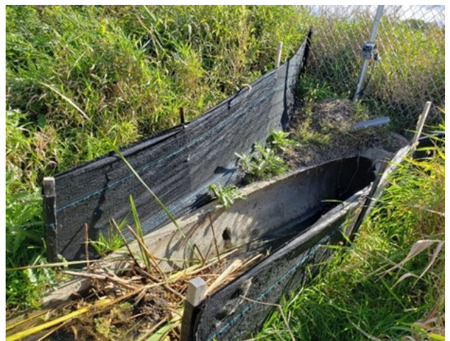
Figure 2. Initial chain-link fence treatment sites. Top: Site preparation and installation of posts and wrap-around end treatments. Middle: Completed chain link fence and end treatment. Bottom: left- MnDOT signage, right- silt-fencing to guide animals into culvert opening.
