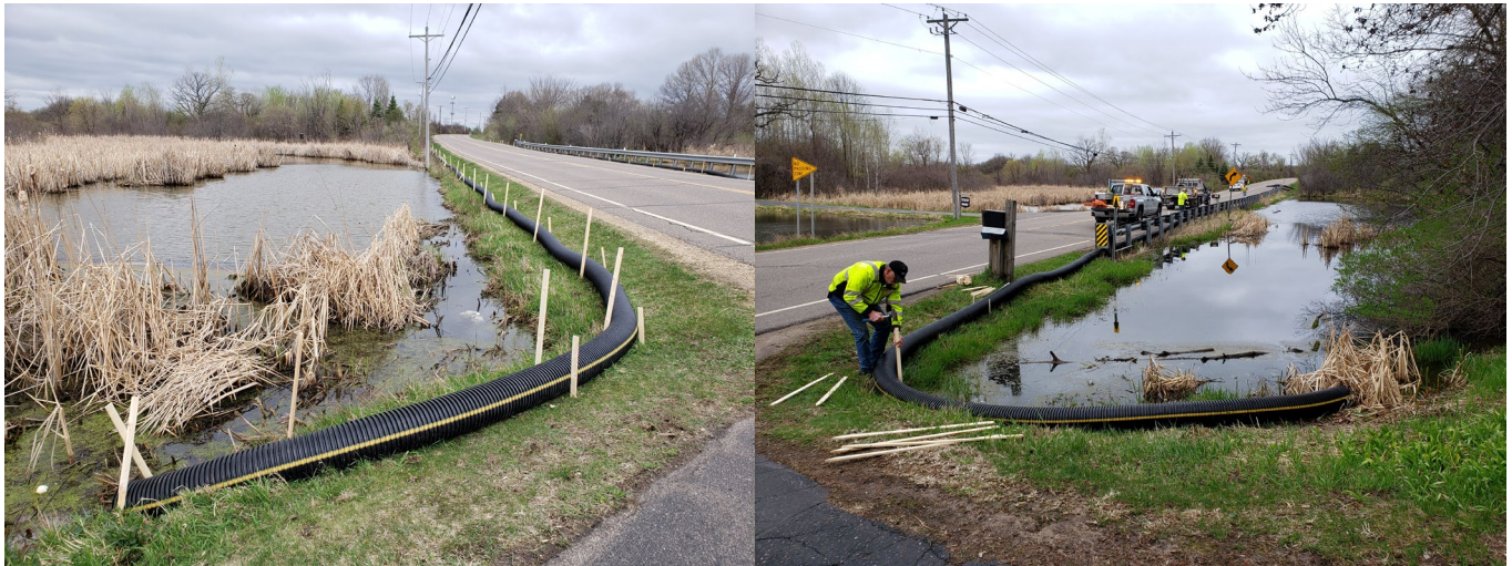
Figure 4. Construction of new 8-inch pipe barrier in Dakota County to keep turtles and other small wildlife off roadways.
