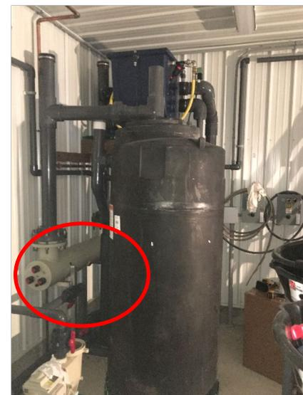
Images 5 (left) and 6 (right): (5) Drum filter installed on wooden shelf (circled in yellow); water reservoir (black tank; left of drum filter); and construction of initial propagation and research system. (6) Ultraviolet sterilizer unit (circled in red), which is located behind the water reservoir, cleans intake water from the Zoo's A lake.
