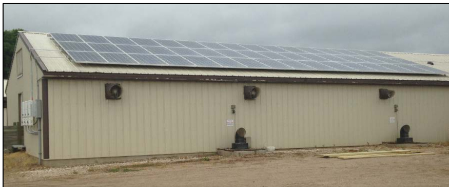
Figure 3: Heliene 60M280 Solar PV System Mounted on the Roof of the WCROC Swine Barn.
