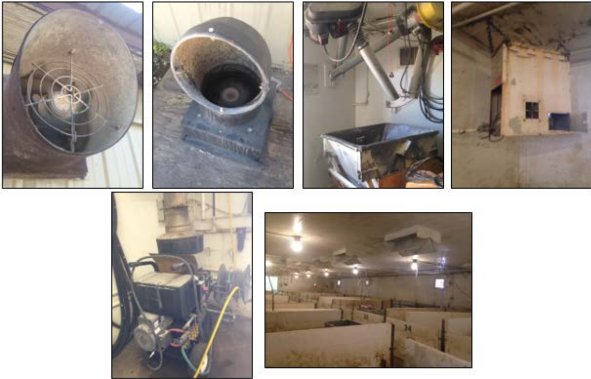
Figure 2: Devices with high electricity requirements at the WCROC finishing barn. From top left, a wall ventilation fan, a pit fan, feed augers, and a heater. From bottom left, the power washer/power washer vent fan and lights.
