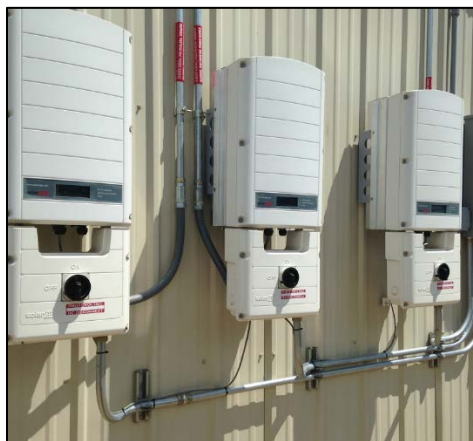
Figure 4: SolarEdge SE9K Three Phase Inverters on the WCROC Swine Barn.
