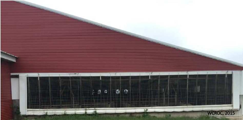
Figure 3. An example of a tunnel-ventilated pig barn with ventilation fans on the far end and an inlet curtain on the near end.
