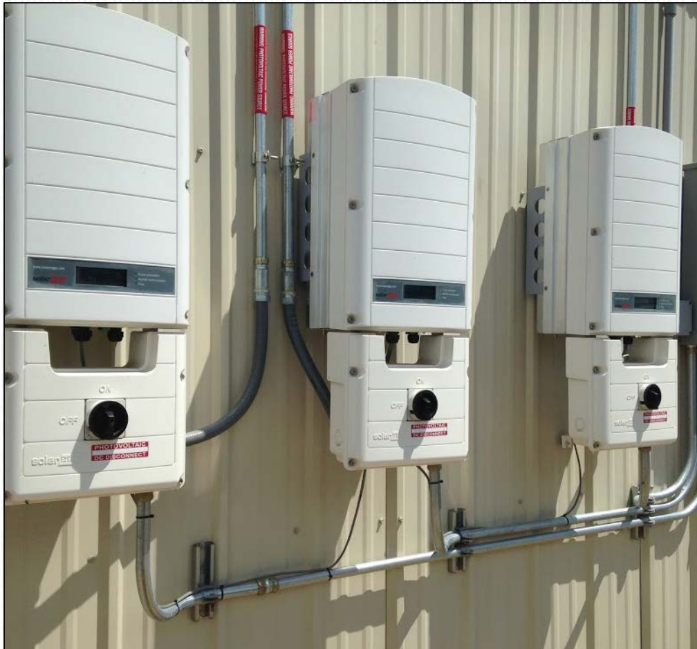
SolarEdge inverters
