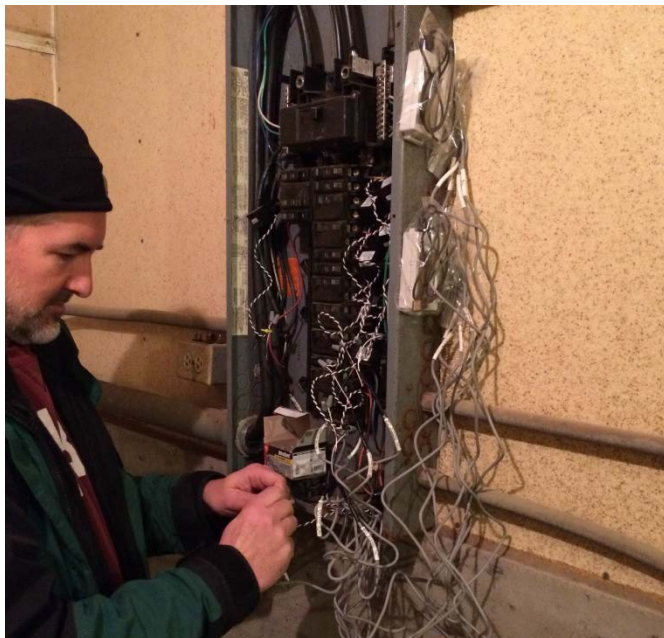
Picture 1. Data loggers being installed in circuit breaker box at a commercial finishing barn
