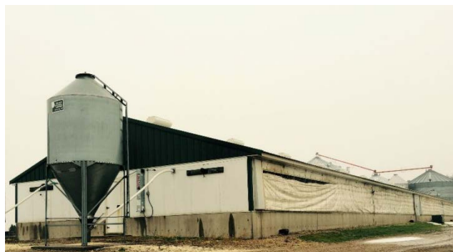
Figure 2. An example of a curtain-sided pig barn.
