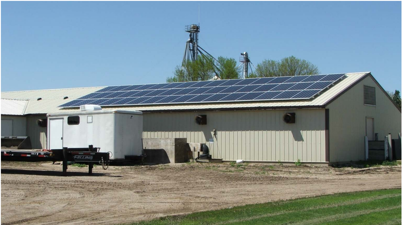
Picture 4. 27 kW Solar PV System on WCROC Swine Facility – East Side
