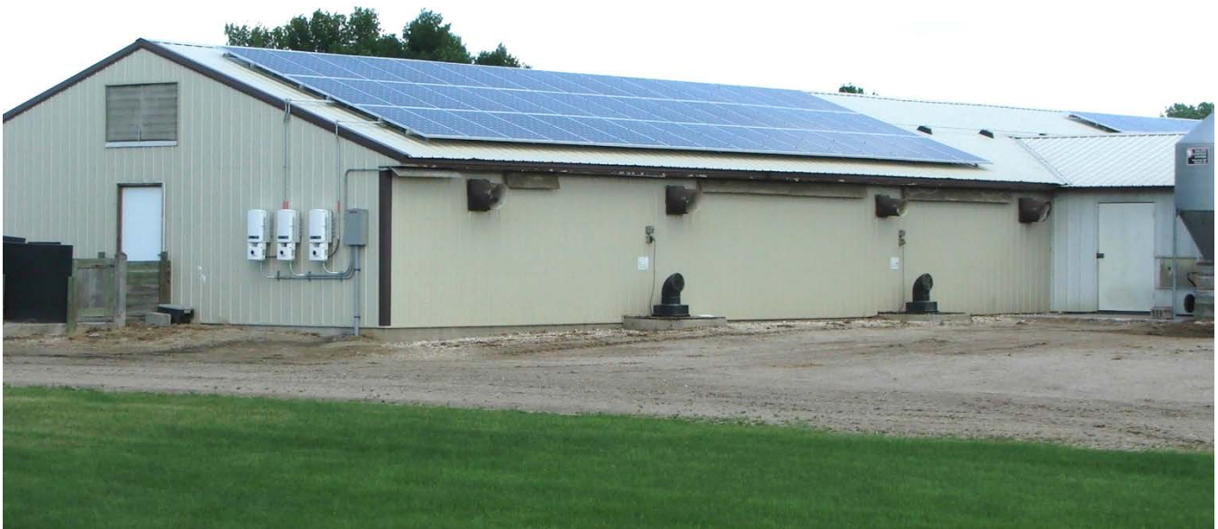
Picture 3. 27 kW Solar PV System on WCROC Swine Facility – West Side
