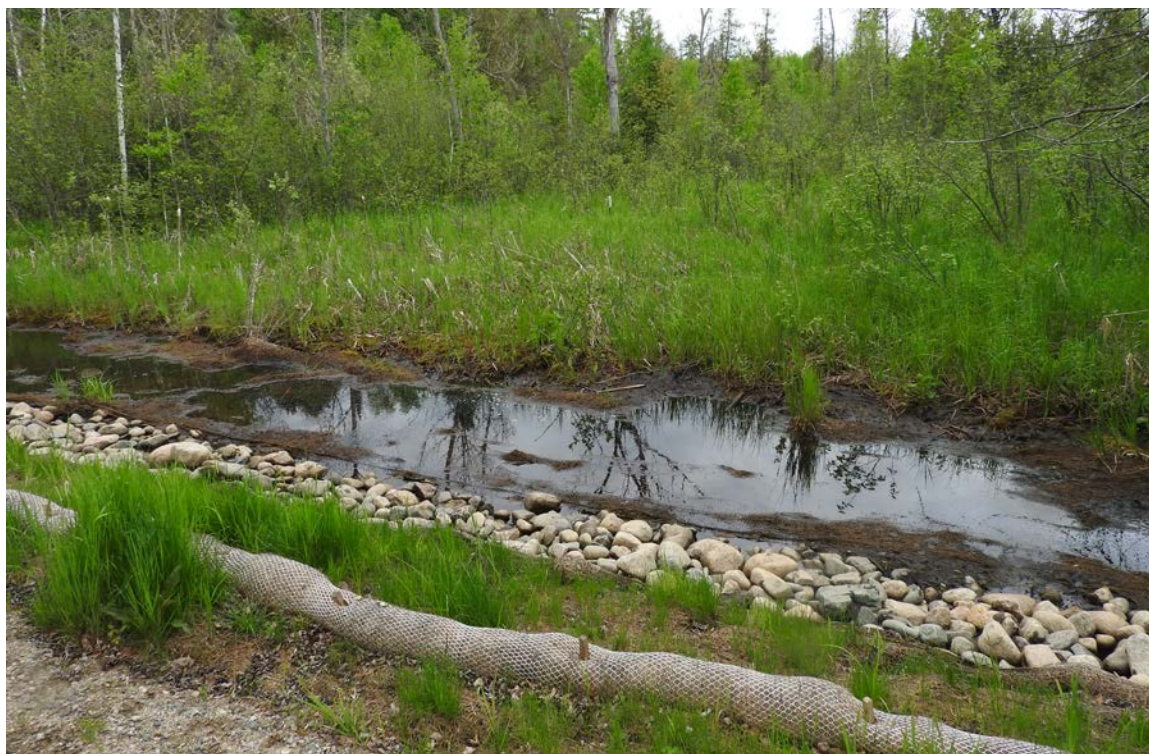
Figure 47. Upgradient of Wirt road after restoration showing lower ponding of water.
