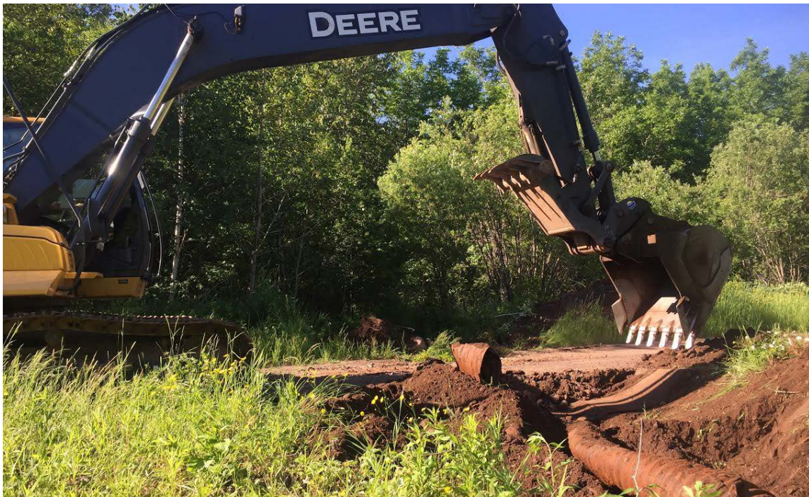
Figure 43. Replacing old culvert at Defrense Road.
