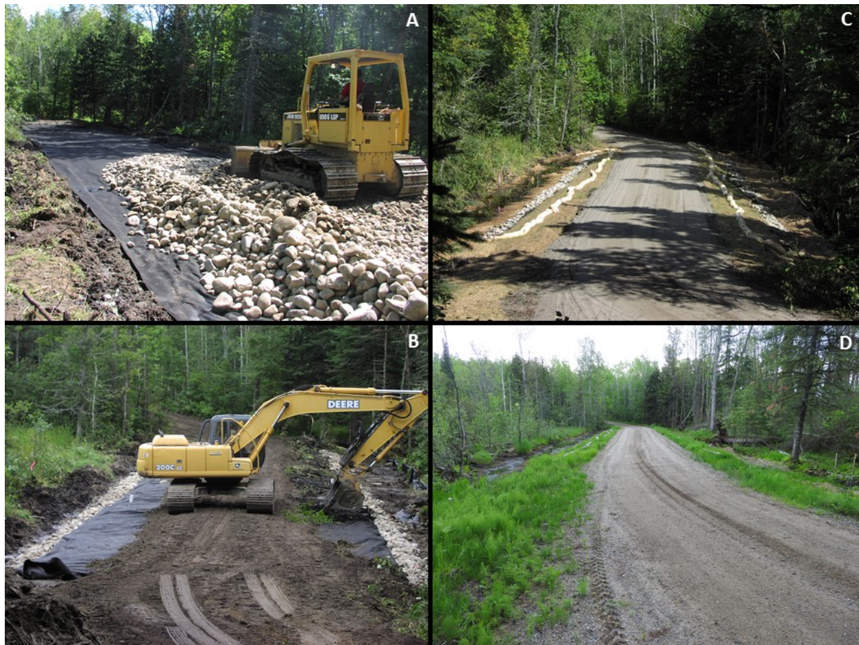
Figure 40. Sequence of Wirt road restoration: A) Roadbed was removed, then geotextile was laid out and 12” of 4 to 6-inch rock was spread out over the fabric, B) then another layer of geotextile fabric and more dirt was laid over the top of the rock, C) additional rock was placed at the toe of the slope over the geotextile fabric exposed below the gravel roadbed and erosion blankets were placed to cover the disturbed surfaces alongside the road, D) finished road as of June 2017.
