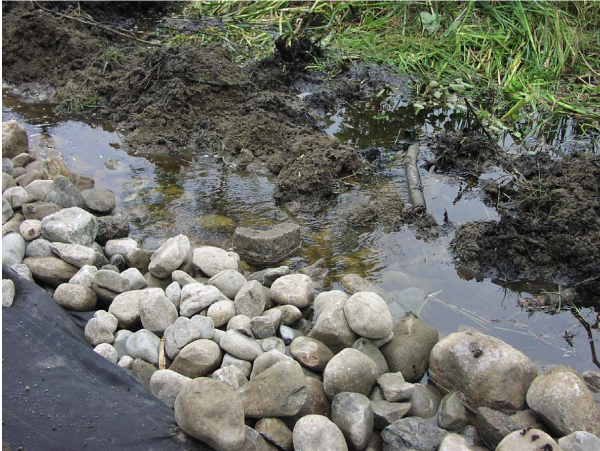
Figure 48. Downgradient of Wirt Road showing water flowing out of the porous roadbed.
