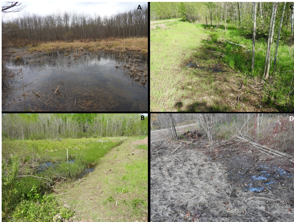
Figure 41. Sequence of Defrense road restoration: A) Upgradient road before restoration showing deep ponding, B) Upgradient road after restoration show large drop in ponding and new vegetation growing, C) Downgradient of road after restoration, and D) Close up of water seeping out under the road on the downgradient side of the road after restoration.
