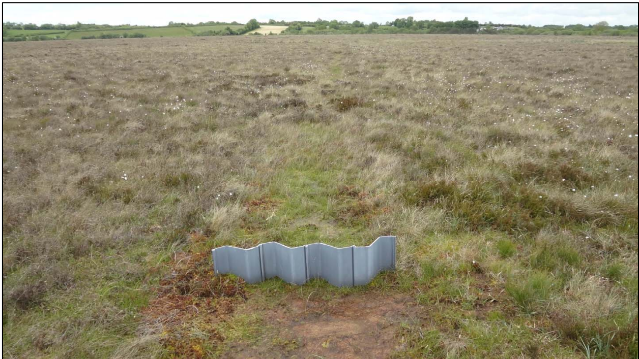
Figure 4: Small ditch blocked using vinyl sheet piling on a restored bog in Ireland. June 2015.
