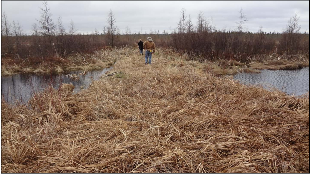
Figure 2: Clay core ditch block at the Brown's Lake Peatland Restoration site. May 2014.
