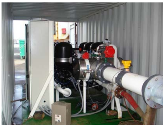
Photo 2 - Hyde Guardian System As Used for Emergency Treatment of Ship Lift Barge "Lucky Angel" in Puget Sound (Hyde Marine, 2009)
