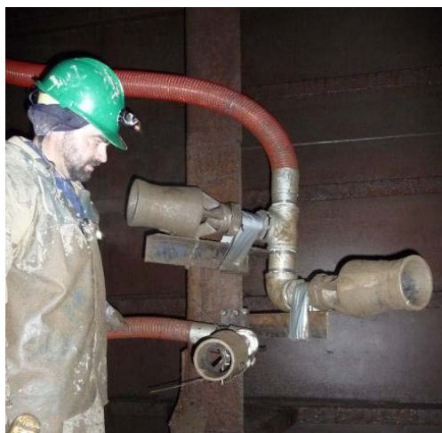
Photo 5 - 45° nozzle setup (lower nozzle part of parallel setup)
