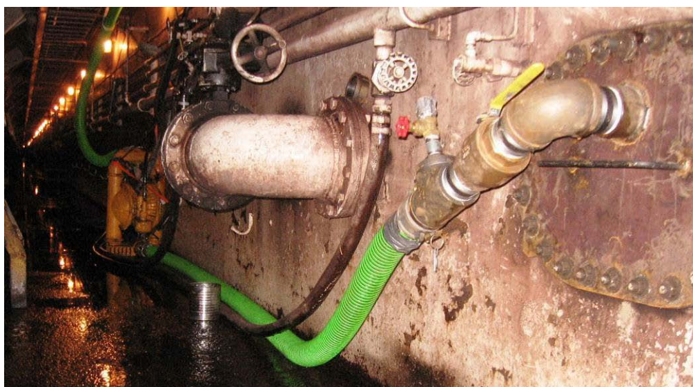
Photo 21 - Chemical injection manifold tee fitting shown, transfer pump in background
