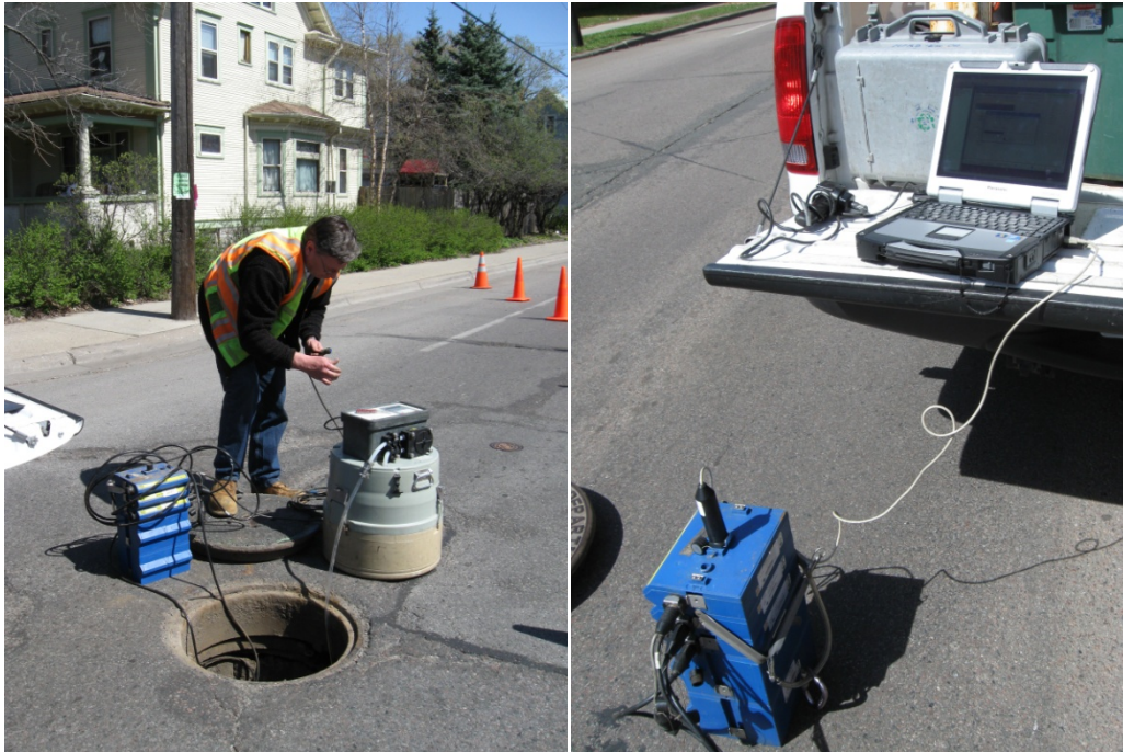
Figure 3. Flow and Water Quality Monitoring Equipment
