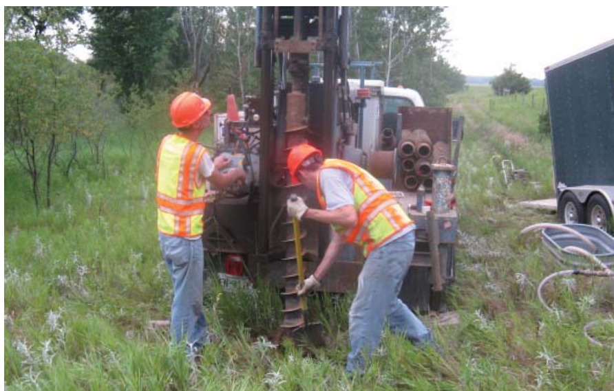
FIGURE 3. Installing a shallow GWLM well using a hollow stem auger drill.
