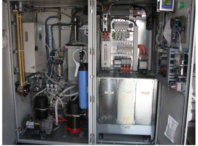
Picture 2. Interior of the electrolyzer.
