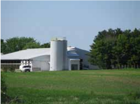
After barn expansion and digester construction.
