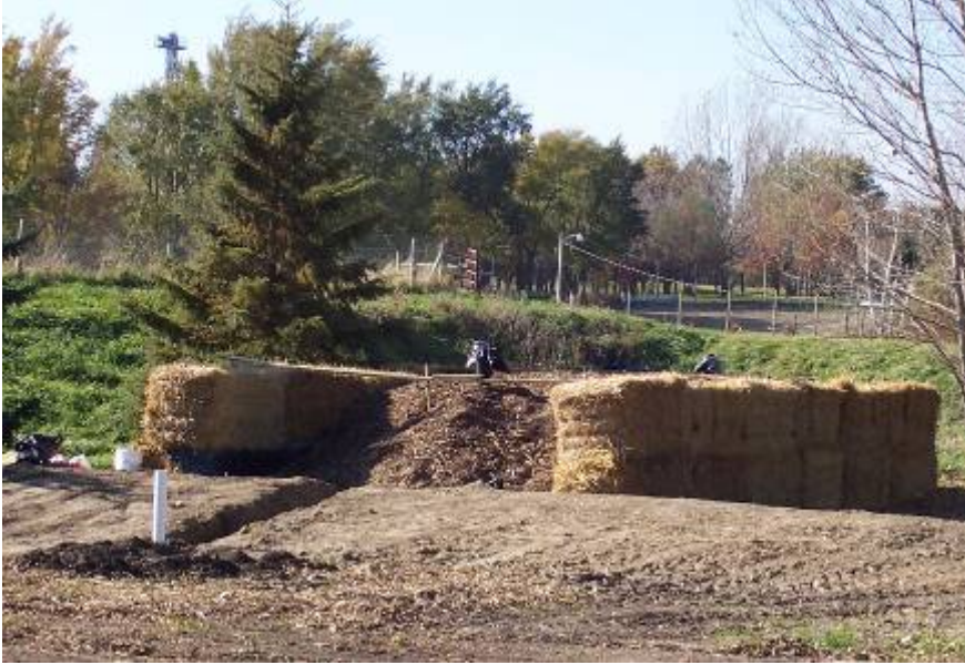
Figure 35: Completed biofilter installation
