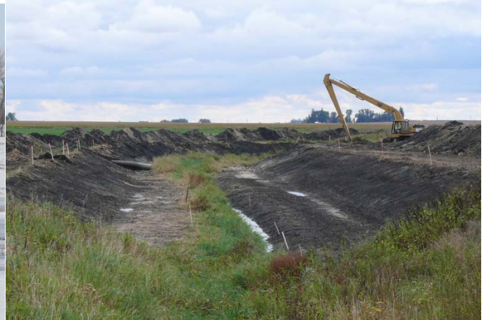
Two-stage ditch hydrology/nutrient mitigation
