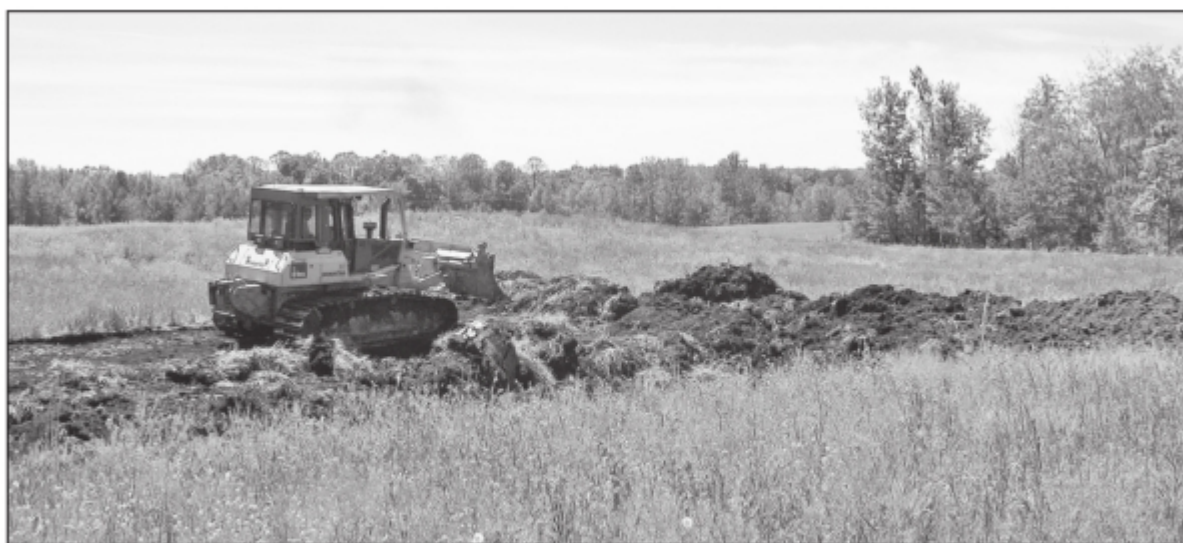
Wetland restoration work can be time-consuming and expensive. In the case above, sediment was removed from a former wetland, and existing tile was removed.
